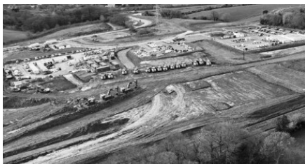
The North Portal construction site
