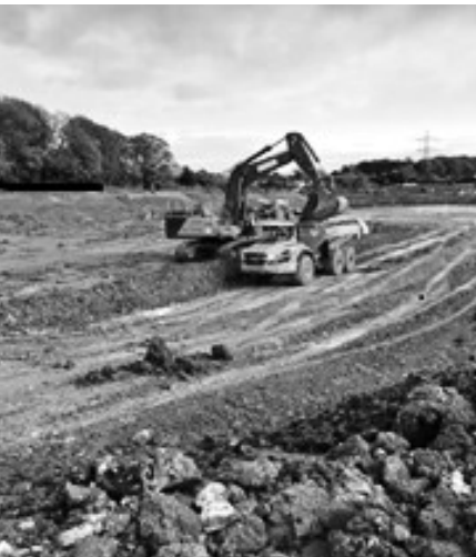
Excavating the cuttings
