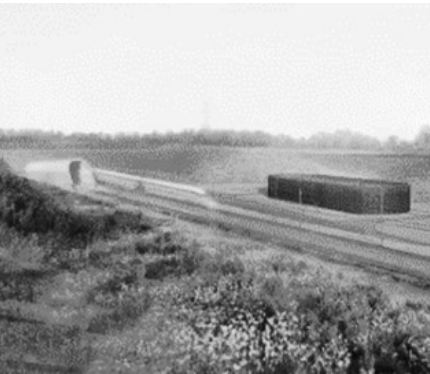
Chiltern tunnel North Portal
