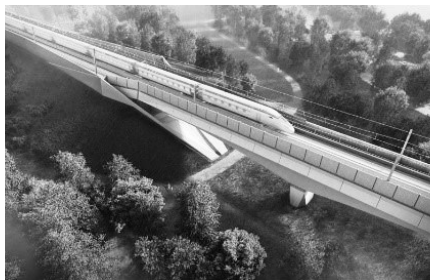
Colne Valley Viaduct (HS2 design)
