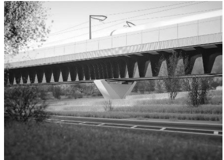
Small Dean Viaduct (HS2 design)
