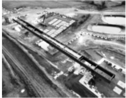
Wendover Dean Viaduct construction)
